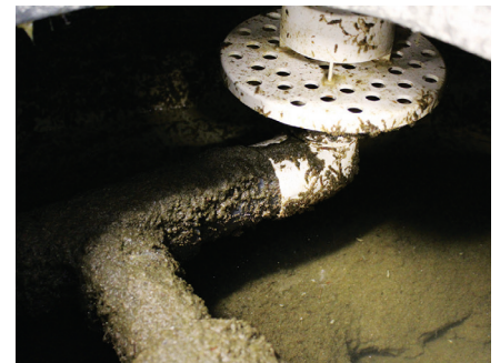
A combination of algae, dissolved waterfowl diet and bacterial film had resulted in the sand in the sand filters loading up rapidly and clumping together.
