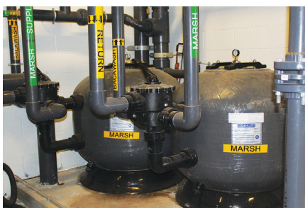
Waterco's Micron Commercial Fibreglass Filters are made from continuous strands of high quality fibreglass filament wound under controlled tension to create a seamless, impervious vessel.
