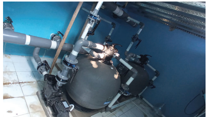
Powering Pristine Pools: A behind-the-scenes look at Tropikana Water Park's cutting-edge Waterco filtration and pumping systems, ensuring crystal-clear waters and uninterrupted fun for all visitors
